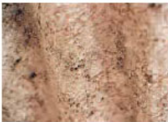
Sprayed coatings on ceiling walls, beams/columns
