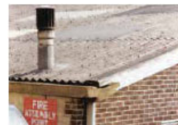
Asbestos cement roof
